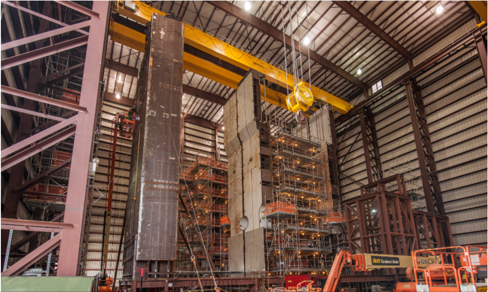
Assembly of part of the Vogtle Unit 3 CA-01 module.
