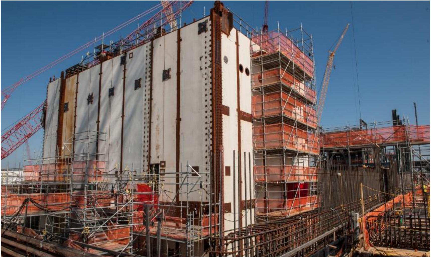
CA20 module inside Vogtle Unit 3 nuclear island.
