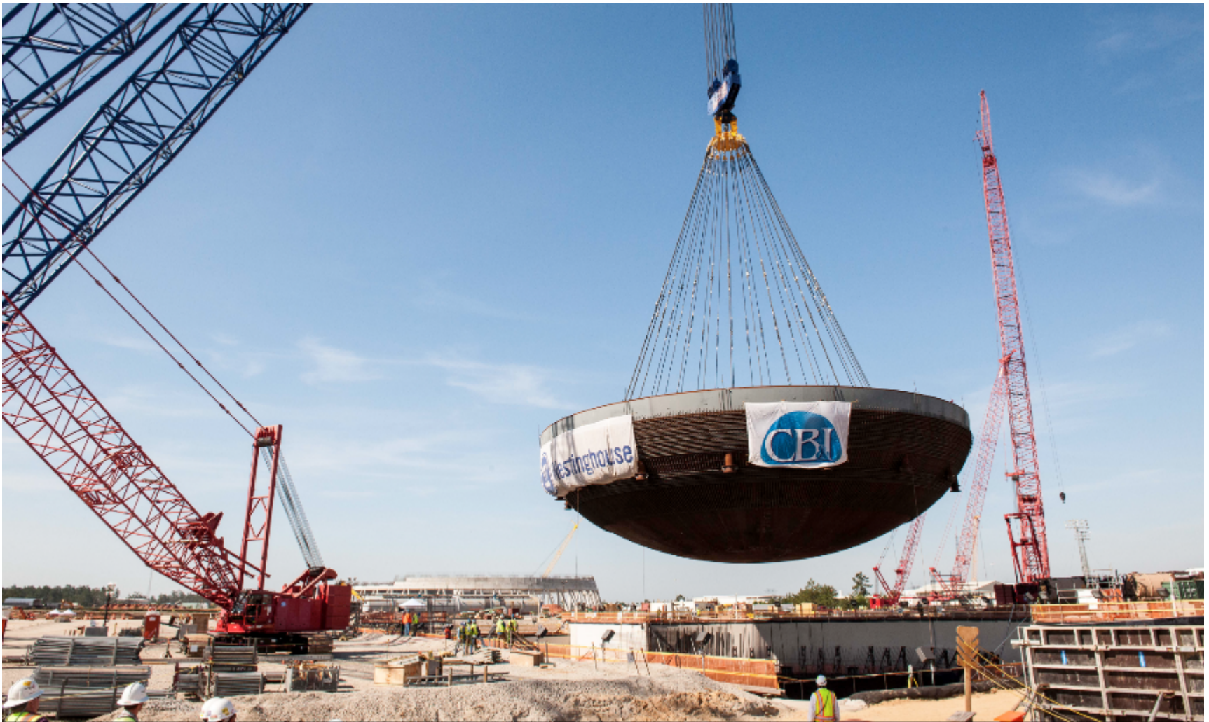
Placement of the Vogtle Unit 4 containment vessel bottom head in the nuclear island.
