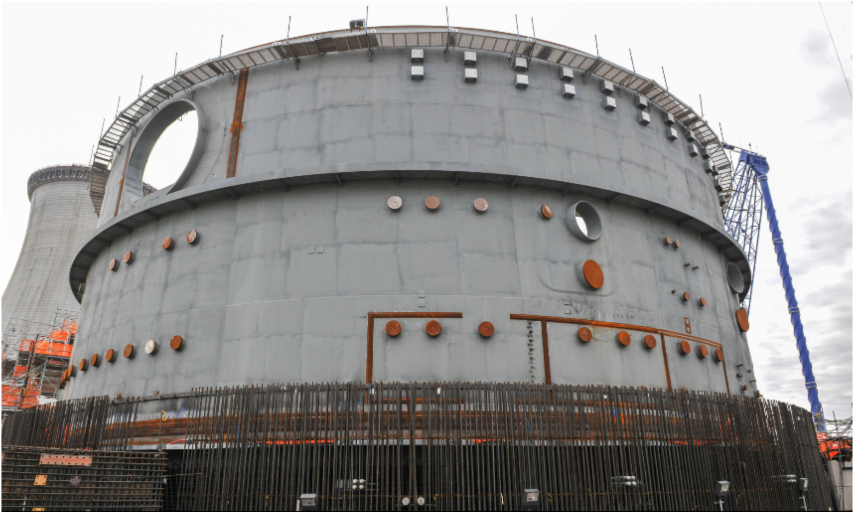
Vogtle Unit 3 containment vessel in the nuclear island.
