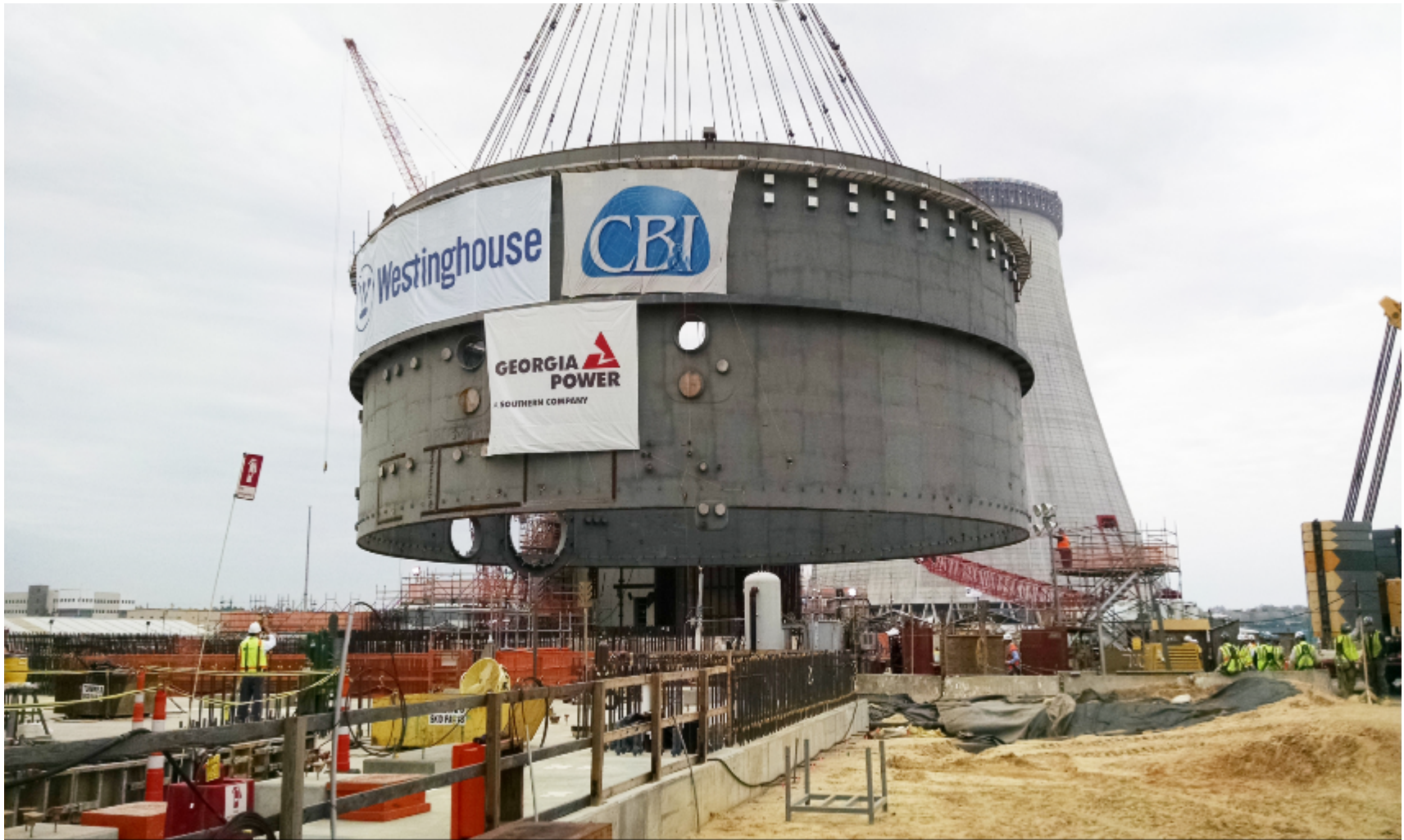
Vogtle Unit 3 lower ring placement
