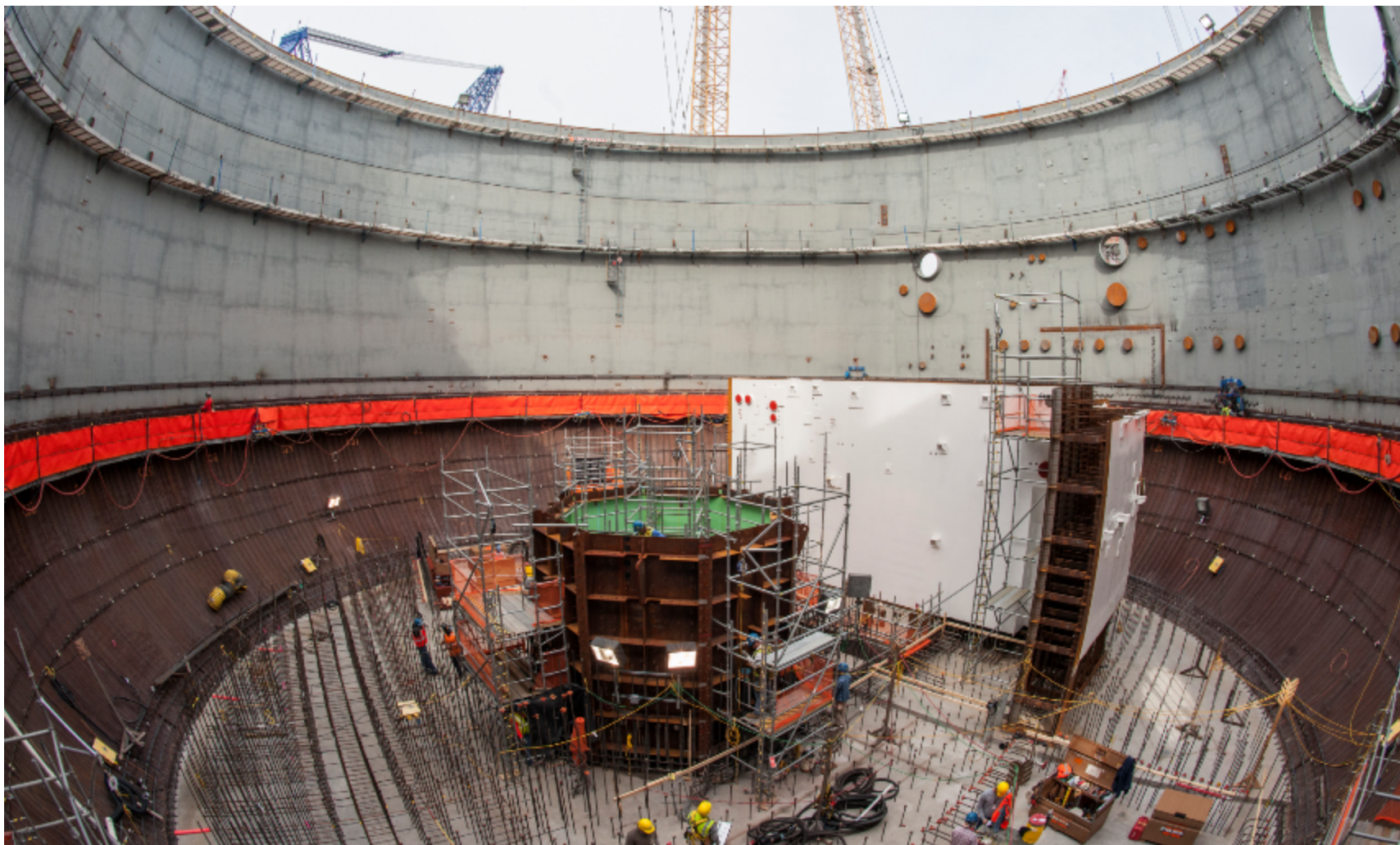
Modules CA-04 and CA-05 inside the Vogtle Unit 3 containment vessel lower ring.
