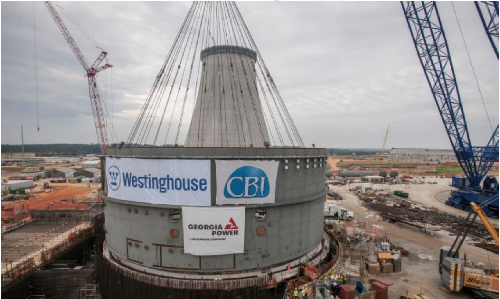
Vogtle Unit 3 lower ring placement
