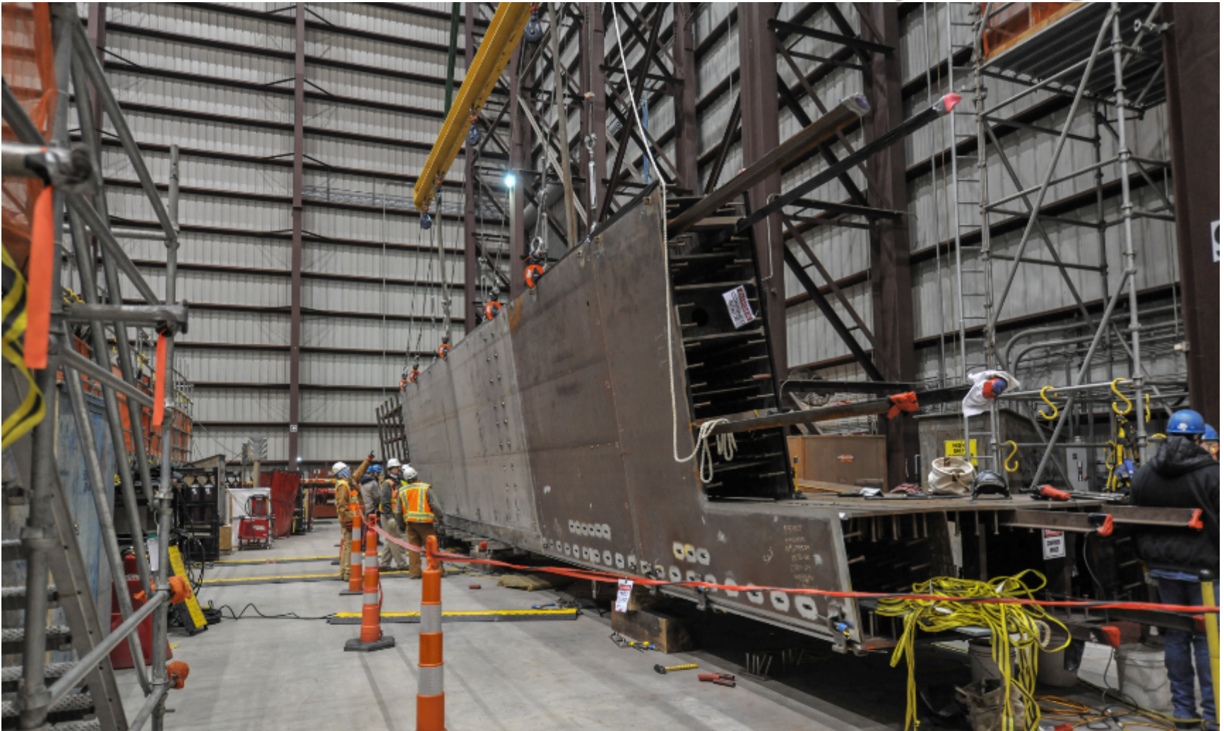
Vogtle Unit 3 CA01 sub-module inside the Module Assembly Building.
