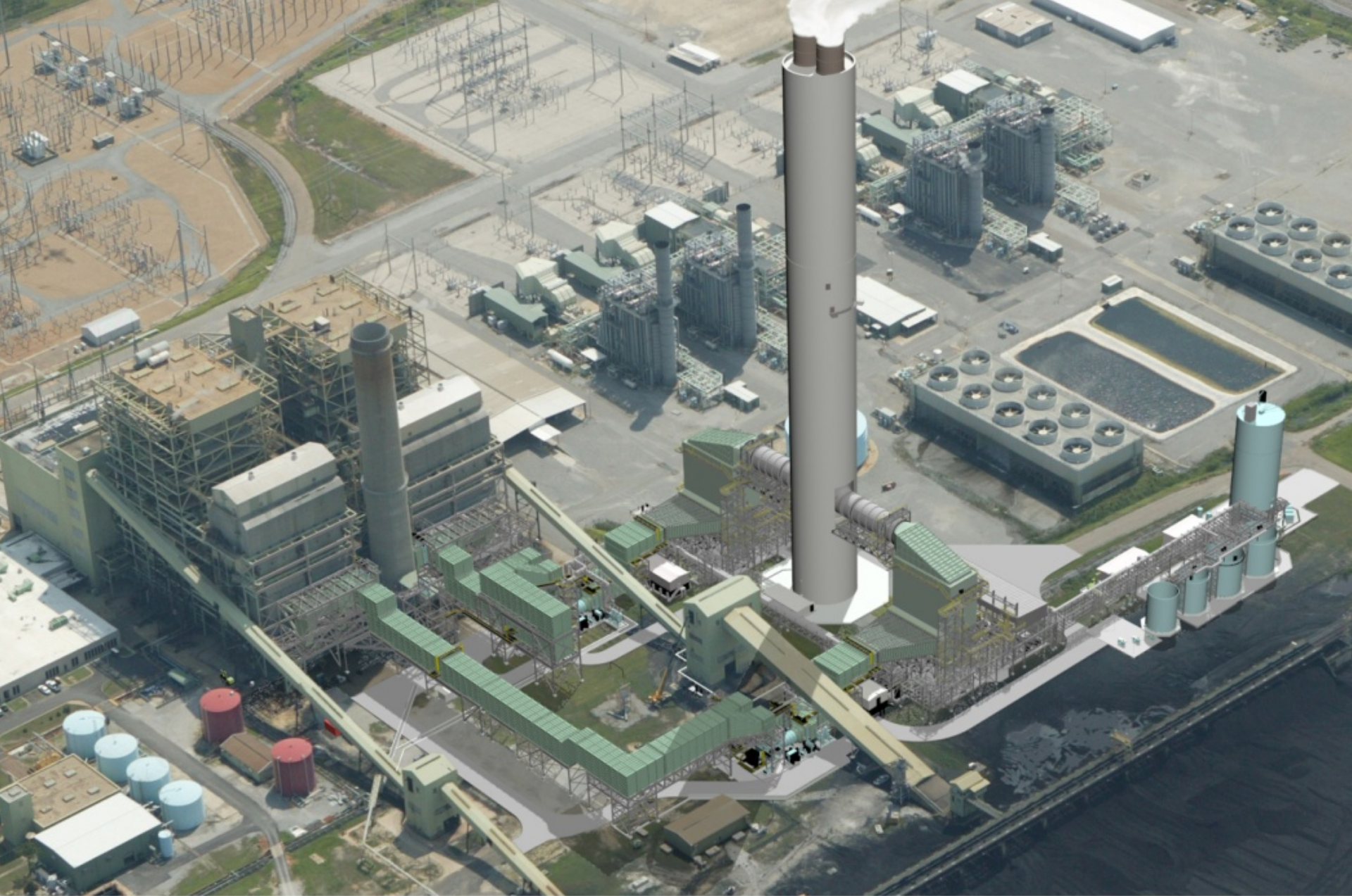
MPC PLANT DANIEL SCRUBBER PROJECT
